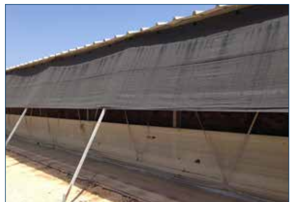
Figure 9. Porous window shades block direct sunlight from entering the house, but allow air to pass through.
